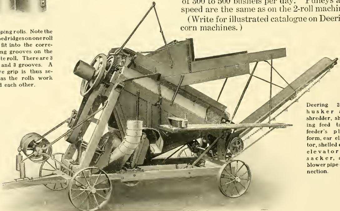
Deering 2-roll husker and shredder, showing feed table, feeder's platform, ear elevator, shelled corn elevator or sacker, and blower pipe connection.
